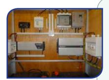
**PV 2 kWp** PV modules ISTAR (IT) Solar charge controller Steca (DE) and Western & Co (IT) - Inverter Studer (CH)
